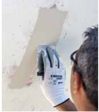
Fairing any defects
