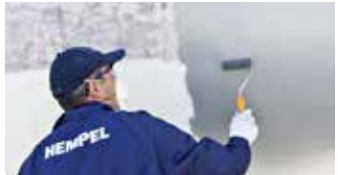
Apply Hempel's Underwater Primer onto prepared surface
